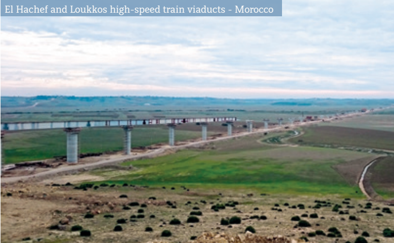
El Hachef and Loukkos high-speed train viaducts - Morocco
