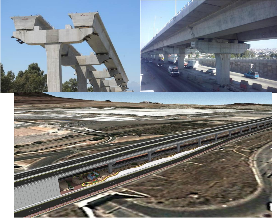
Figure 3: The structure during construction phases and with isolators already installed
