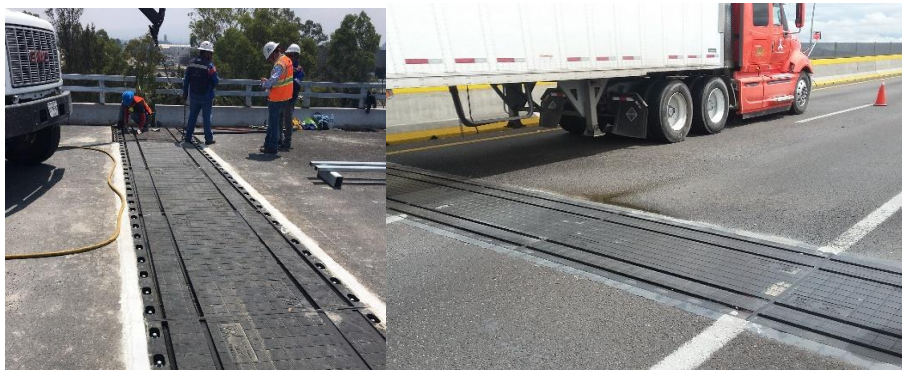
Figure 7: Expansion joint during and after installation
